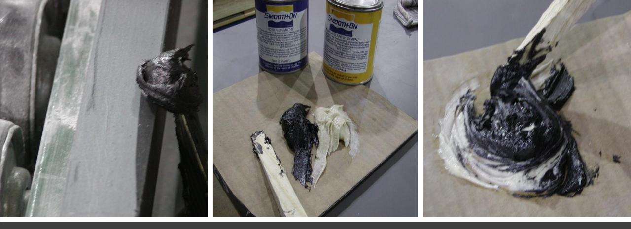
Mix Smooth- on and Fill the chip or broken Piece make sure to mix the Smooth On correctly 50/50 ratio.
