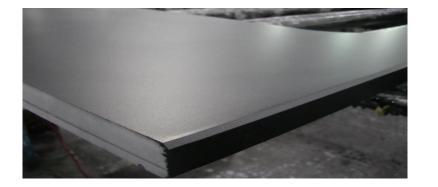
In most cases a small amount of paint will get on the surface of the counter top after painting the edge. Be sure to remove excess paint from top surface using a rag with lacquer thinner. In doing so be sure not to remove paint from beveled edge.
