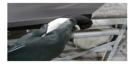
Than after the edge has been sanded proceed to paint the edges that have been sanded. Make sure you follow Epoxy Edge Paint Mixing Instructions below.
